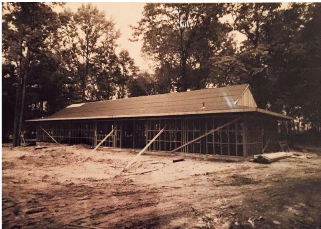
The Old Orchard Swim Club under construction in the mid-1960s.
