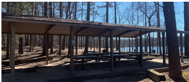
Clerk of Course (existing pavilion)
