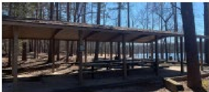
Clerk of Course (existing pavilion)
